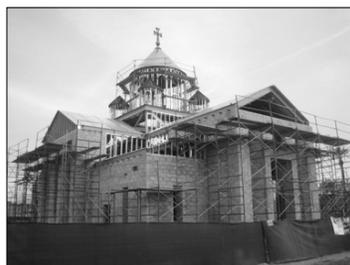
The construction of the Armenian Apostolic Church of the Desert is on schedule. During the month of February, the interior metal stud framing was completed and is ready for pre-wiring. Fire Sprinkler lines now run throughout the building and plumbing lines will be installed and connected soon. The 12' front door framing has been powder coated and installed, in preparation for the finished double arched metal doors. A final decision on the exterior stone veneer has been made and will soon be
